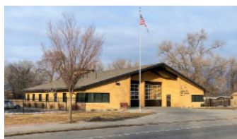
Ogden Fire Station #4
